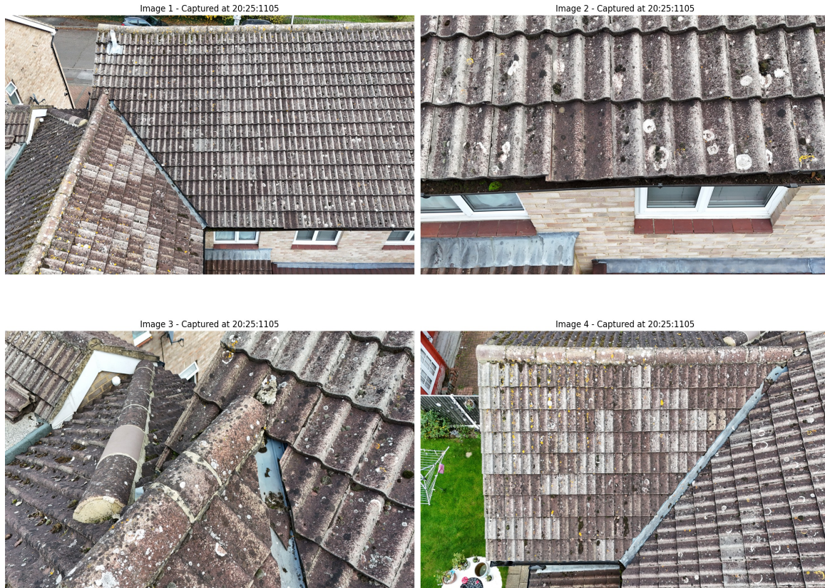
Figure 1: Overview of captured aerial imagery showing all four survey positions
